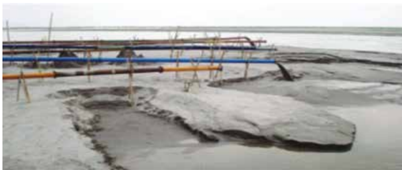
Figure 1: Dredging operations at riverbeds of Jamuna river in Bangladesh [5].
