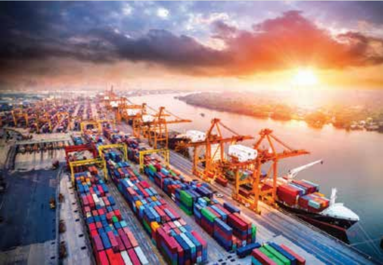
Smart and deep-water ports, efficient shipping and logistics industries will be instrumental for the development of the Blue Economy
